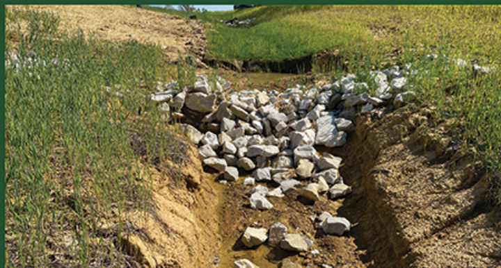
Fully vegetated InstaTurf vs Rock Riprap in Channel
