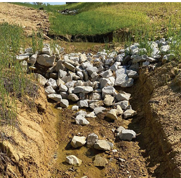
ShearForce10 installation in channel vs rock riprap.
