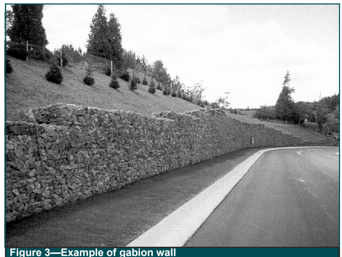
Figure 3—Example of gabion wall
