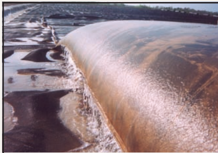
Water draining from a Geotube® container.
