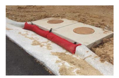
The Big Red filter is a REUSABLE inlet protector that prevents sediment from leaving the jobsite during construction. There are no pockets to fill, no velcro bags, and no assembly is required. Simply place Big Red in front of the inlet, making sure it lays in the contour, and you are DONE!
