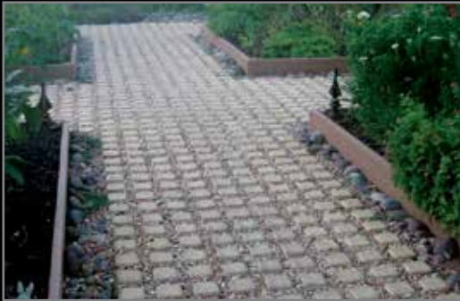
AGGREGATE INFILL
