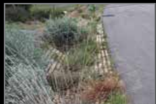
DRAINAGE SWALES
