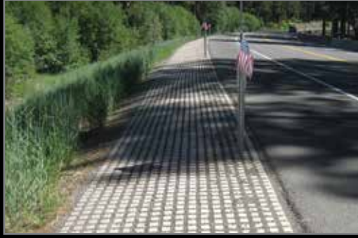
AGGREGATE INFILL
