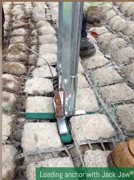
Gas powered driver installation.
