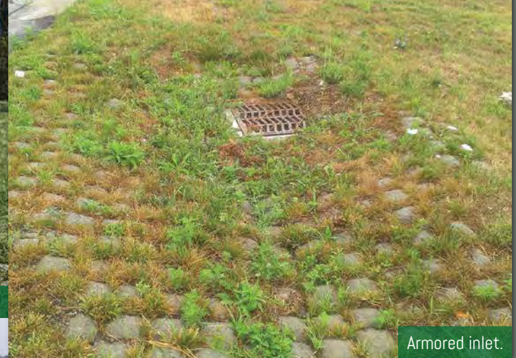
Outlet armored with Flexamat®, 3 years after installation.
