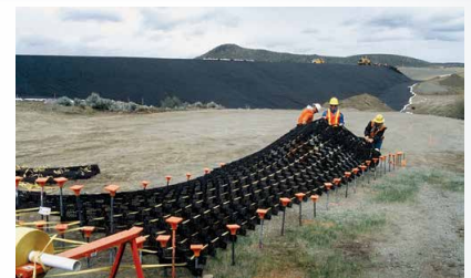
GEOWEB® tendon anchoring system
