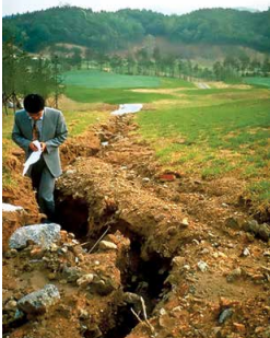
Severe scour in unprotected spillway
