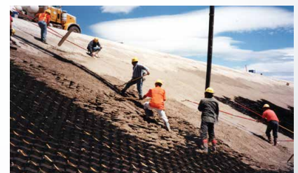
No additional formwork or reinforcement is required
