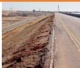
1) Erosion caused by overtopping
