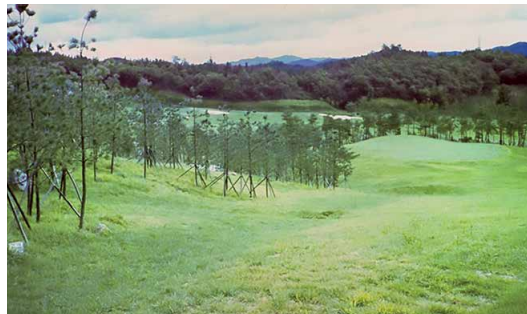
GEOWEB® vegetated spillway repair
