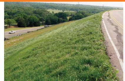
3) Fully vegetated GEOWEB® slope
