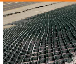
2) GEOWEB® slope erosion repair
