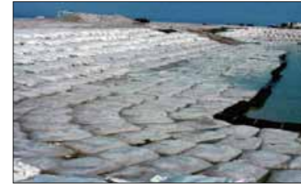
Geobag® revetment construction
