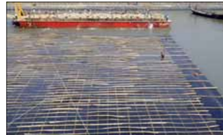
Mirafi® geotextile beneath rock bed protection
