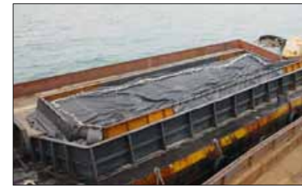
Geocontainer® offshore breakwater construction
