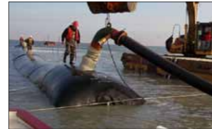
Geotube® containment dyke construction
