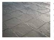
GEOWEB<sup>®</sup> slopes with concrete infill provide economical, hardarmored protection of slopes exposed to severe hydraulic or mechanical stresses. The quality,
