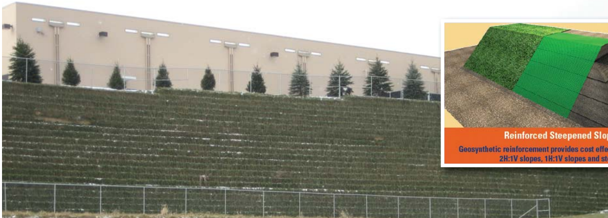
Lowe's Store, Western Hills, OH, Height = 65 1H:3V Miramesh GR inside wire basket wall.
