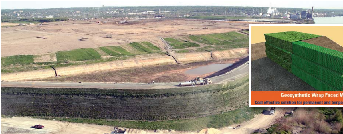
Cherry Island Landfill Expansion, Delaware River, Miramesh GR inside wire basket facing, Height = 75 ft.
