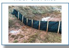
WBSF (woven belted silt fence) addresses the trapping efficiency and stormwater release required for the success of the practice. Five (350 lb.) belts are woven within the fabric, making this silt fence one of the strongest on the market.
