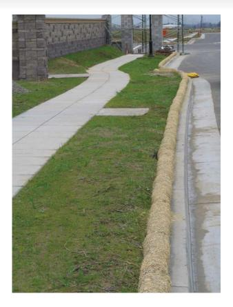
Straw wattles are an effective and economical alternative to silt fence and straw bales for sediment control and stormwater runoff. Straw wattles can be placed and staked along the contour of newly constructed or disturbed slopes. Their use to capture and keep sediment on the slopes is a best management practice (BMP).
